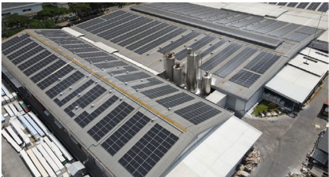
4.47 MWp of solar panels installed at Unit 2 Cikarang
