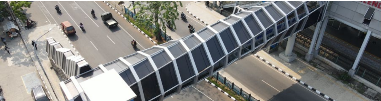
SolarTuff Solid polycarbonate sheet installed at Klender pedestrian bridge
