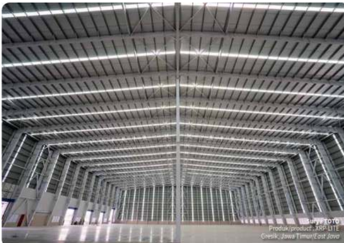
Exhibit 6: Company's product at ceramic plant
