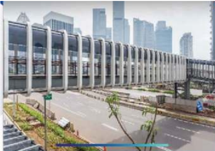
Exhibit 4: IMPC's product at pedestrian bridge in Jakarta
