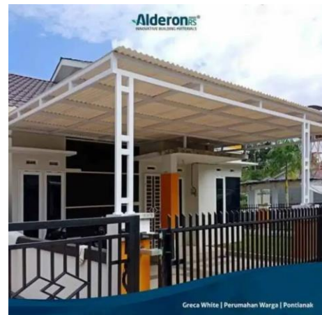
Alderon RS roof
