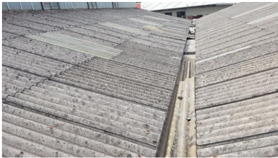
Asbestos Roof
