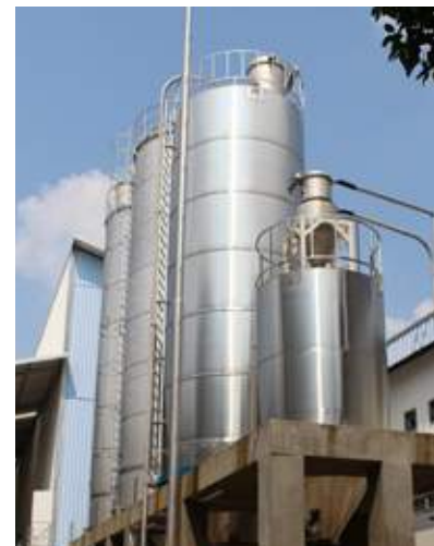
▲ Silo for Automatic Blending and Storage
