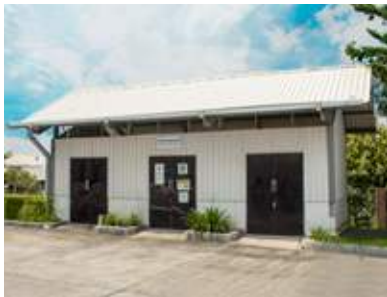
▲ Warehouse for Hazardous Materials
